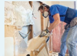
Drywall & Cement Sheets
