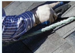
Roof Shingles & Siding
