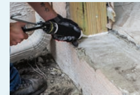
Plaster, Putties & Caulking
